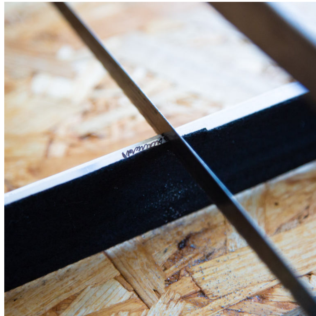
fig.1.10: Cutting of white glue strip at marked position
