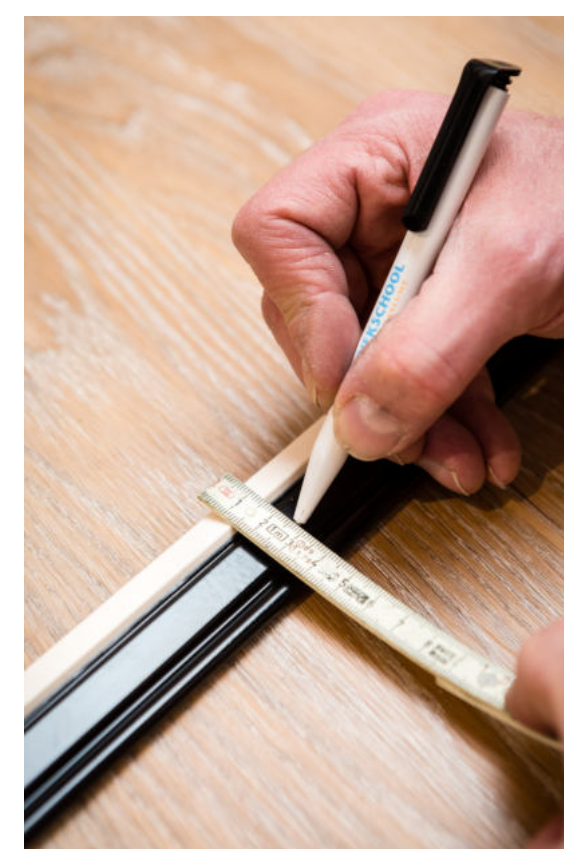
fig. 1.9: Mark cutting/ sawing position for middle bracket
